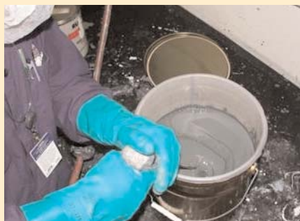
Primer being mixed in 5HD pail liner.
